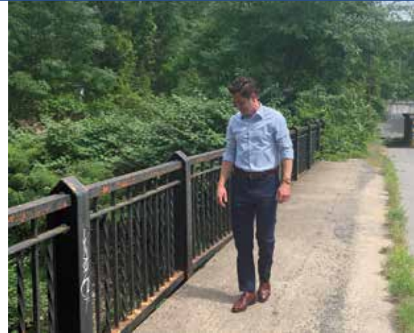
Rep. Mullins inspects crumbling sidewalk on Ash Street Bridge.
